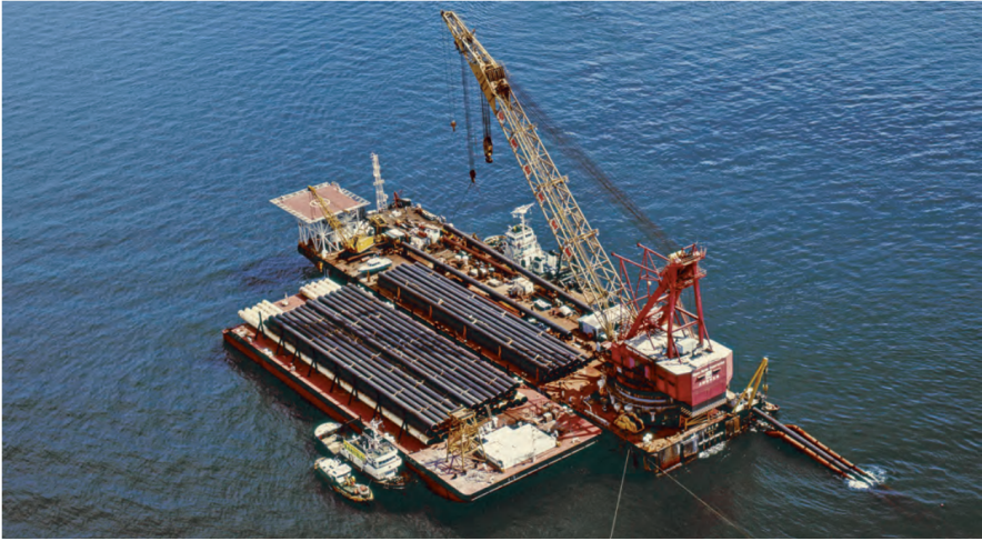
Figure 1: Rig with pipes to be laid [5]
